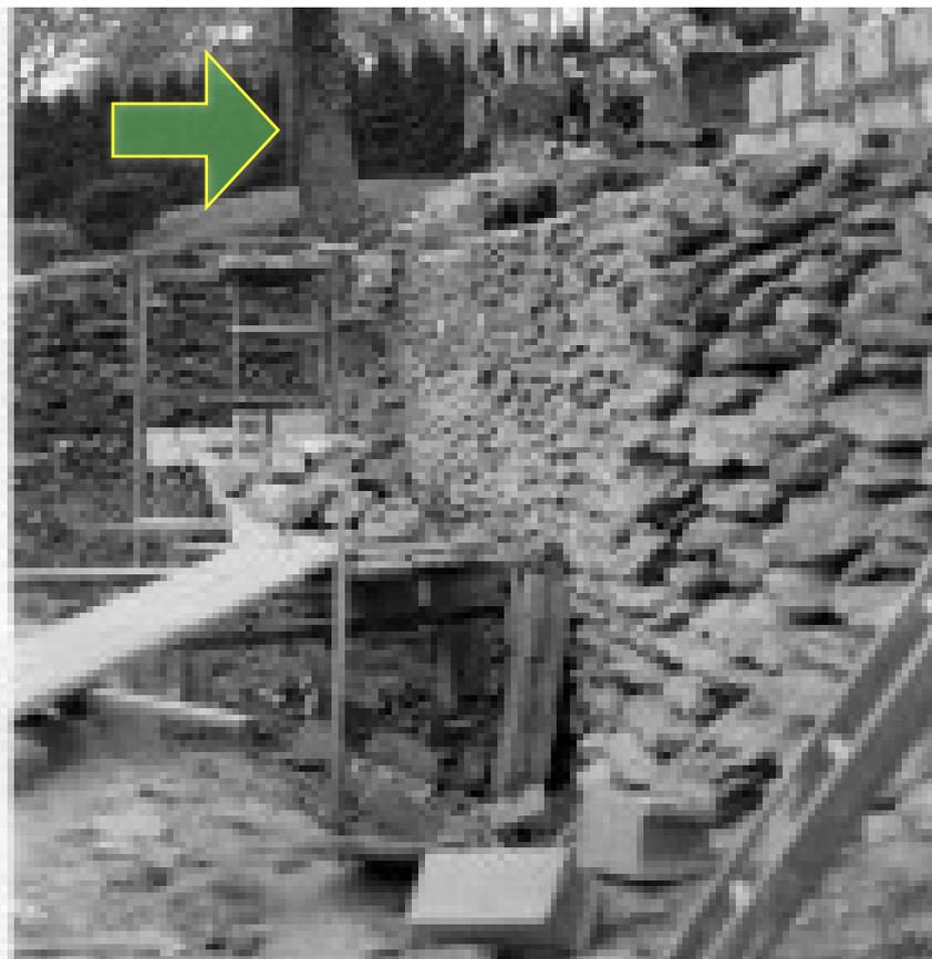
These photos show Hershey's Mill Dam undergoing work to repair and strengthen the spillway, which was damaged by major flooding in 1972. The reinforced spillway was refaced with the original stones to maintain the dam's historic look. Note the tree to the left of the spillway, which is also visible in the preceding photo. The fact that the tree was not removed demonstrates that only a small (albeit significant) portion of the dam was affected by this work.
